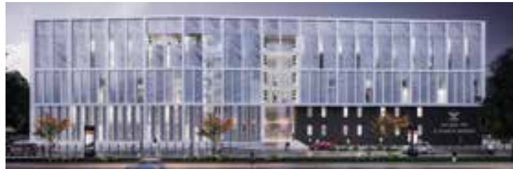
TCDD Scada Center, Ankara
