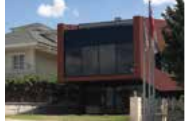
31/23 Commercial Building, Ankara
