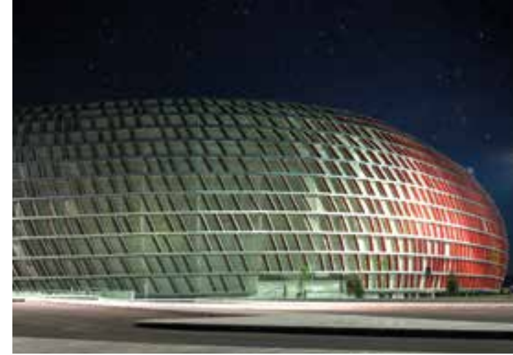
Gaziantep Stadium - BKA - 2017 - Gaziantep
